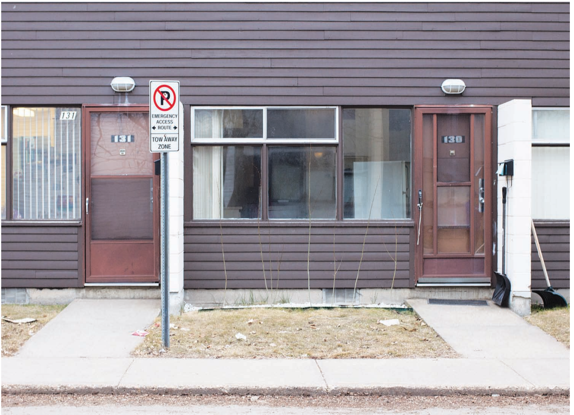
MOULD IN MICHENER Unit 130 in Michener Park (above) has been vacated due to the presence of mould. The following page shows photos of Unit 131 (top left, bottom left) and Unit 130 (top right, bottom right). CHRISTINA VARVIS
